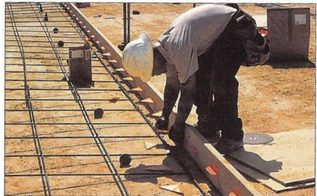
Worker installing diamond plate dowel pocket formers on base supports, which were previously attached to form. Note no form penetrations are required. Note short dowel length and long spacing as compared to typical dowels.
